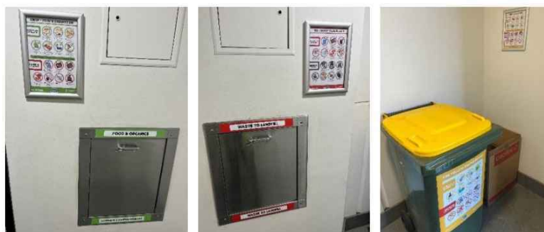
Figure 16: FOGO and Landfill chutes and the comingled recycling bins on each level
