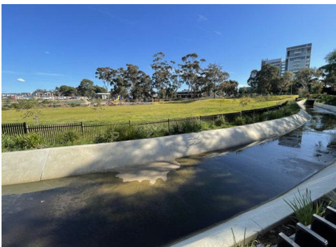
Concrete swale
