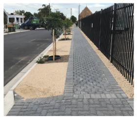
West Torrens Detail Type 1: Permeable Paving
