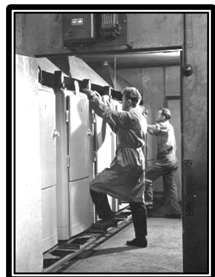
Kelvinator Cabinet assembly line c. 1940. Product M5W. Old factory building fronting Everard Avenue; replaced by two-storey office building c. 1942. Inset – early version of Kelvinator symbol
