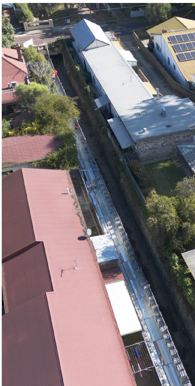
Leah Street to Ethel Street Channel Construction
