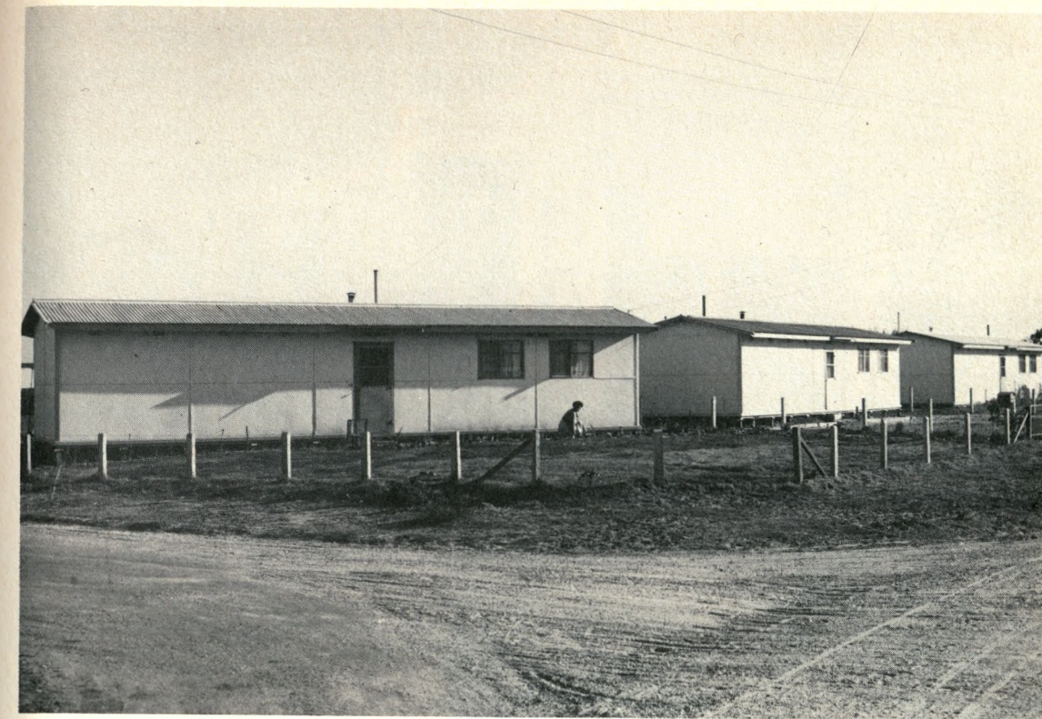
157. These S.A. Housing Trust Emergency Homes at Camden in 1951 were made of timber frame and asbestos sheeting.
