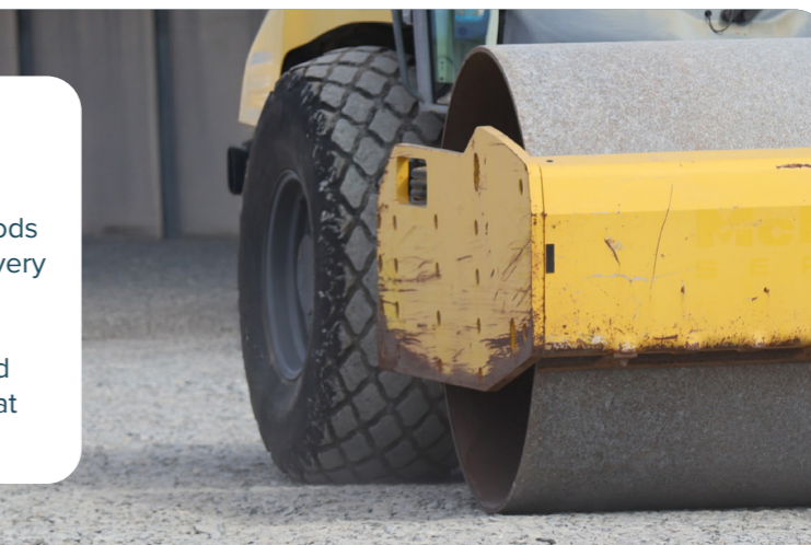
A compaction roller is being used to stabilise the ground
