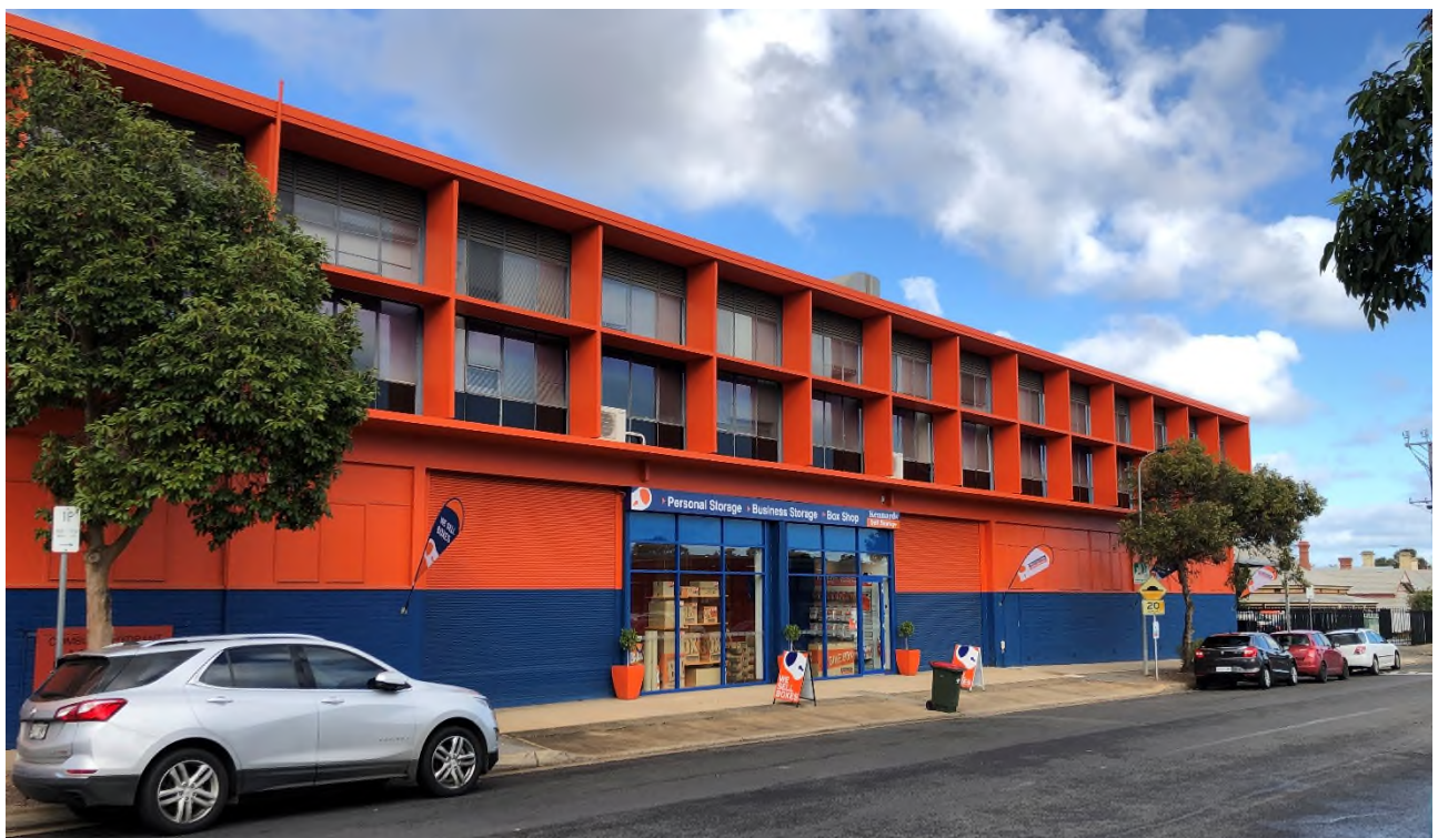
Figure 1 - Subject Site, viewed from Goodenough Street
