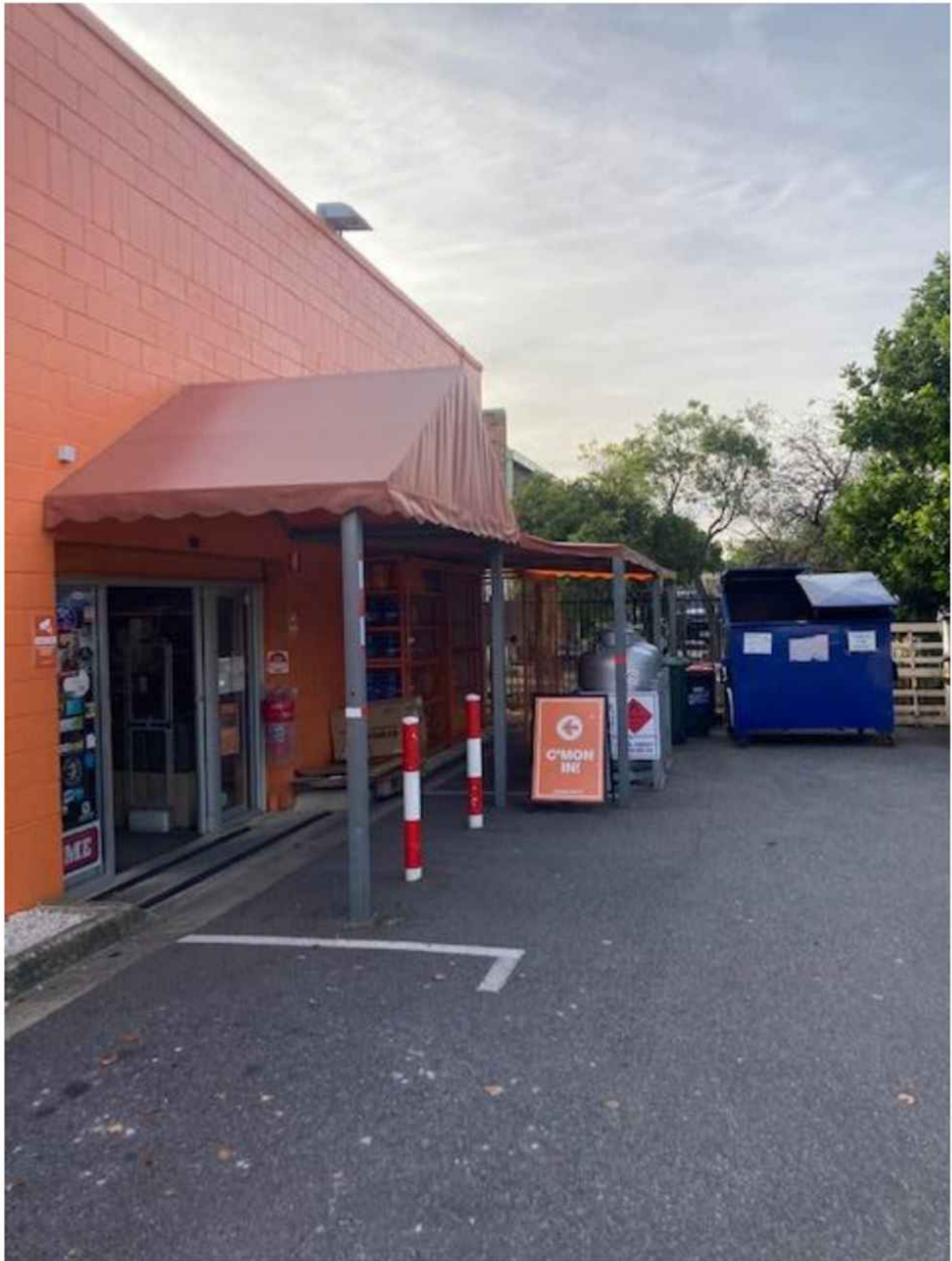
Figure 3: Existing unapproved rear canopies in existing carpark
