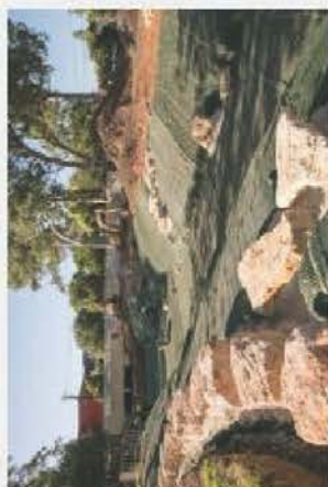
Brownhill Creek Upgrade Pyramat and Stepping Boulders January 2019
