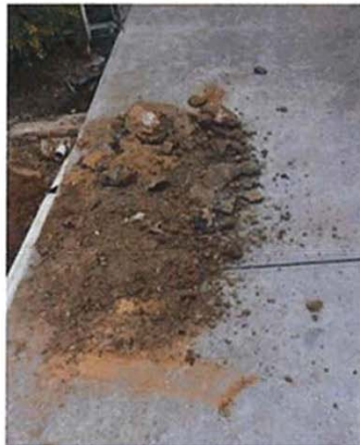
Example of broken bitumen and road base removed ahead of garden planting
