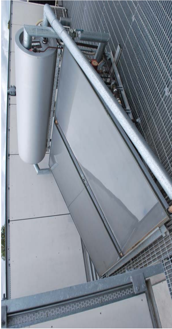
Solar hot water system being used to reduce gas consumption for heating water
