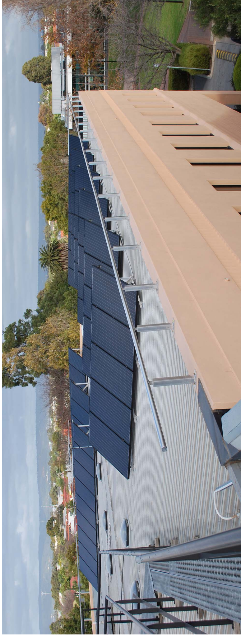
Thirty kilowatt solar panel system on Council's Civic Centre
