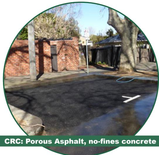
**CRC: Porous Asphalt, no-fines concrete**
