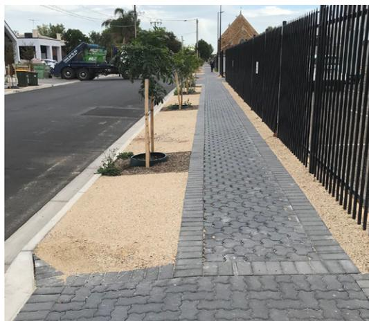
West Torrens Detail Type 1: Permeable Paving
