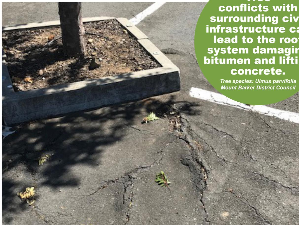
**Tree conflicts with surrounding civil infrastructure can lead to the root system damaging bitumen and lifting concrete.**
