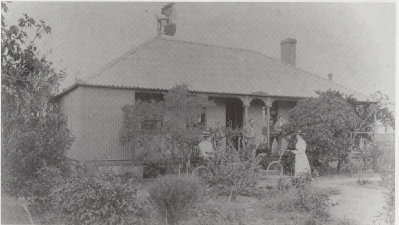
Fig 2. Nathaniel Hone and his family in front of Colonel Light's old home c.1896 (Mortlock Library). Although the original house may not have had a verandah, and would have had a shingled roof, three of the four elegant windows of the two 'large and lofty' front rooms can clearly be seen. The front of Light's house would naturally have looked across his garden and estate to the city he had planned. The remains of a windmill standing above 'Light's well of capital water' can be seen above the roofline.
