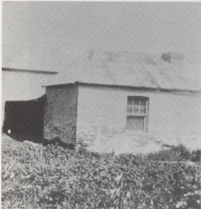
Fig 6. View looking south-west.
