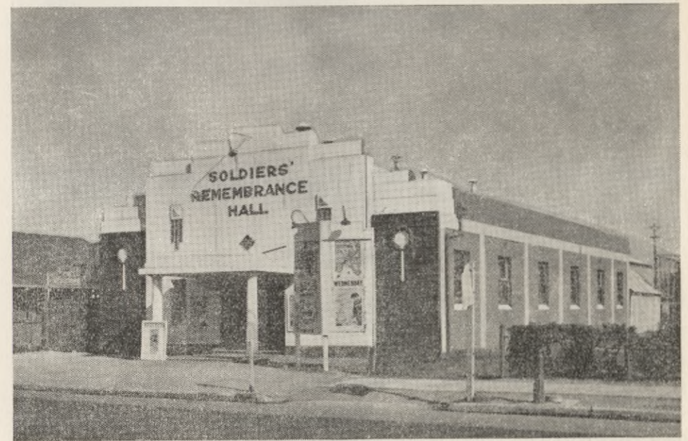
The Keswick & Richmond Sub-Branch Remembrance Hall, South Road, Marleston
