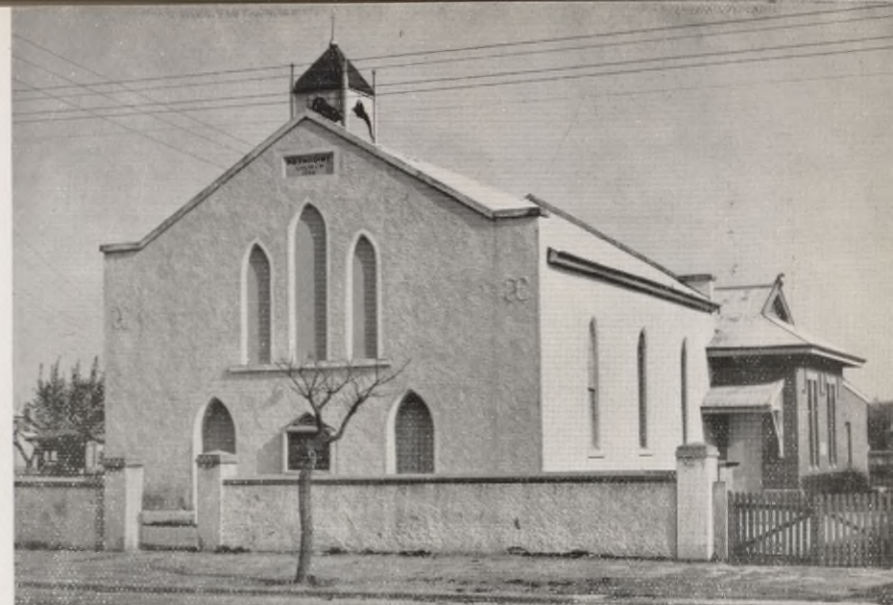
METHODIST CHURCH, MARION ROAD, PLYMPTON.
