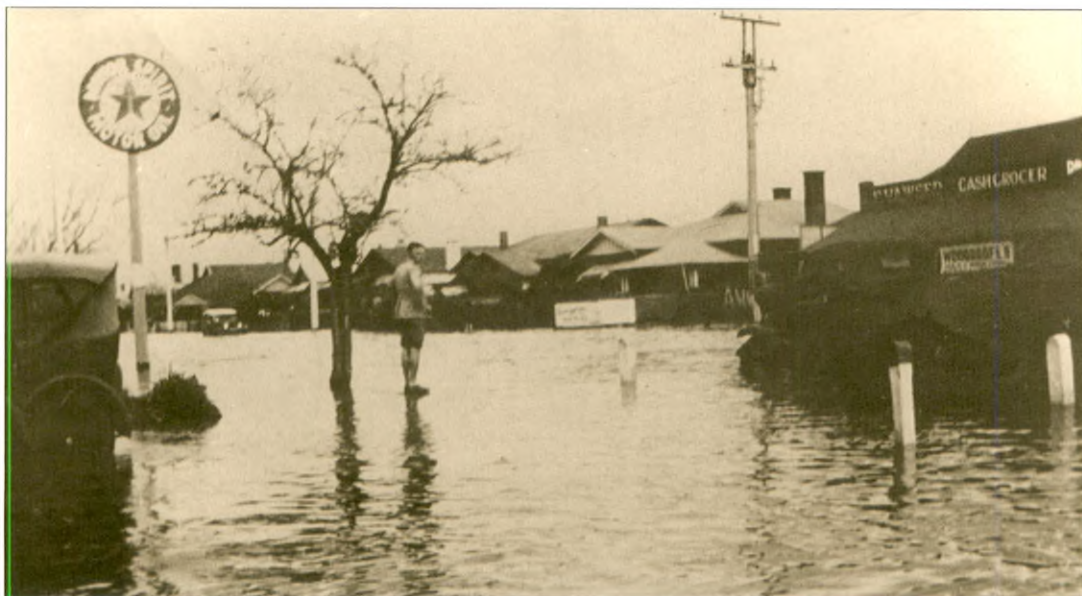
Flooding at the intersection of Henley Beach and Marion Roads, 1932. (WTHS)
