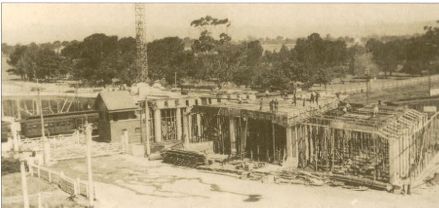
View to the north-east showing the Bakewell Bridge under construction in 1925. (THS)
