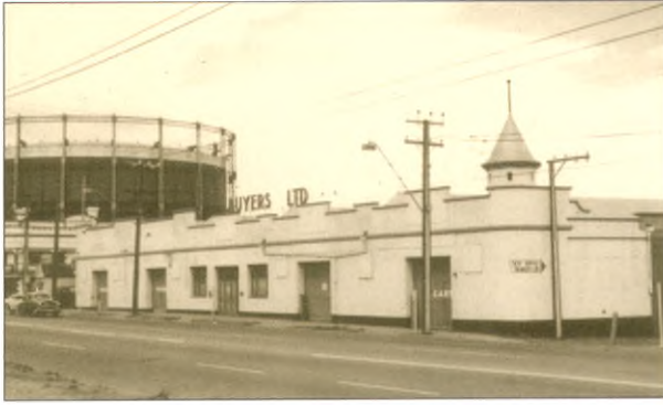
View to the south-east along Port Road c.1960 showing the gas-holder. (THS)
