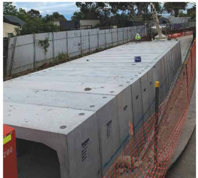
Culvert installation
