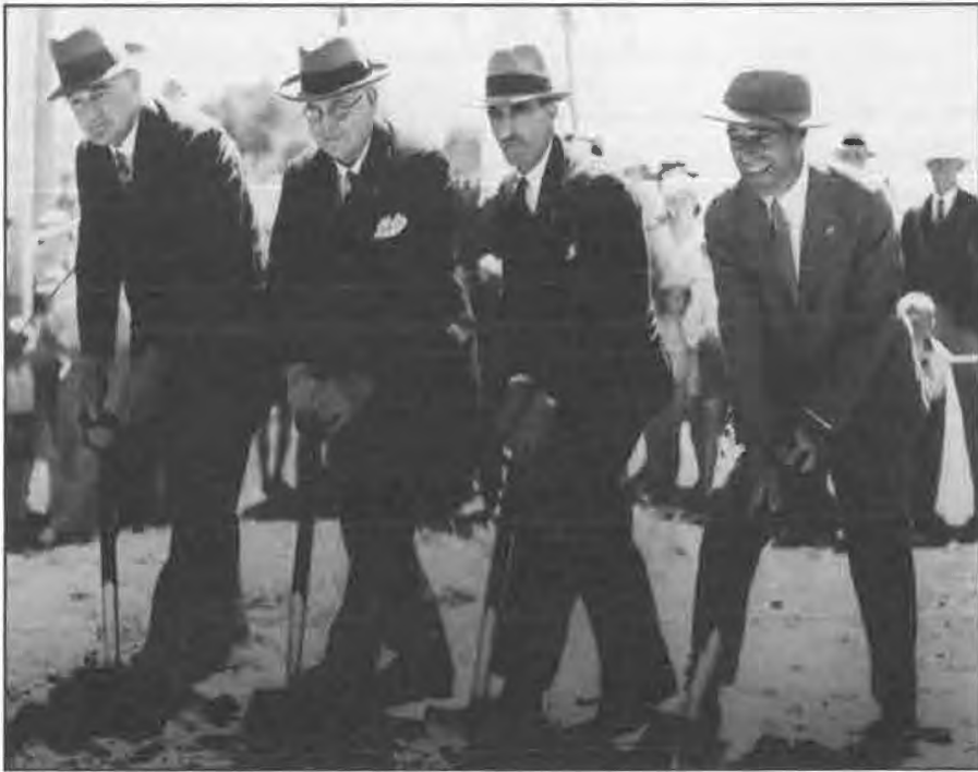
Turning the first sod for beautification works of Anzac Highway, 1 February 1938 (W.T.C.). A.P. Blesing, Minister of Local Government, W. Fisk, Mayor of Glenelg, J. Soutar, Mayor of Unley, A. Chambers, Chairman of West Torrens Council
