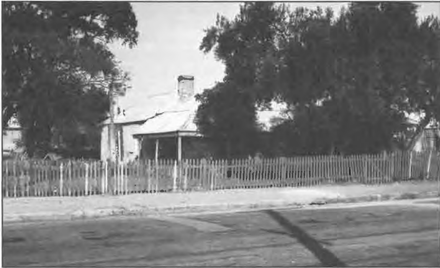
Home of District Clerk John Ruddock on Burbridge Road, Hilton, which for a time also served as the Council offices (W.T.C.)
