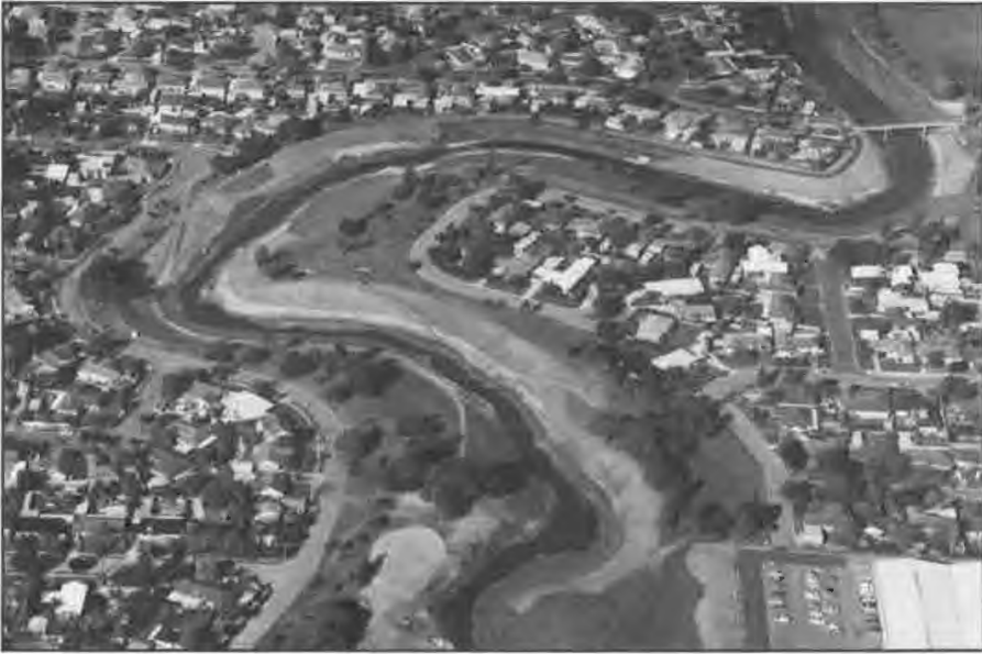
View of engineering works associated with flood mitigation works on Torrens River, 1983 (W.T.C.)
