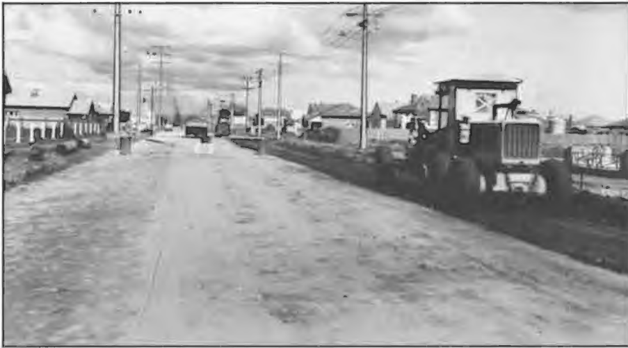
Realignment of Marion Road at Cowandilla, 2 August 1956 (H.D.)
