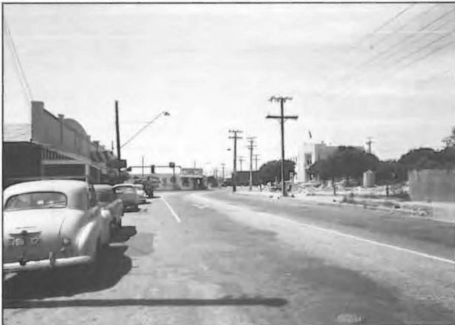
Burbridge Road near Brooker Terrace intersection, looking east, 4 March 1965 (H.D.)
