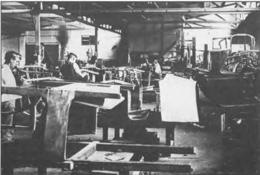
Motor body building at Richards (M.L.)
