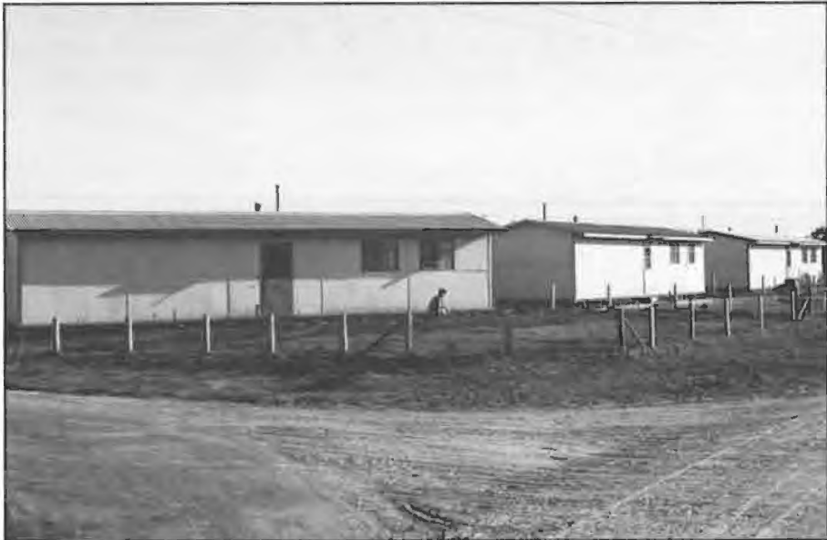
Emergency homes erected by the South Australian Housing Trust at Camden, 1951 (W.T.C.)
