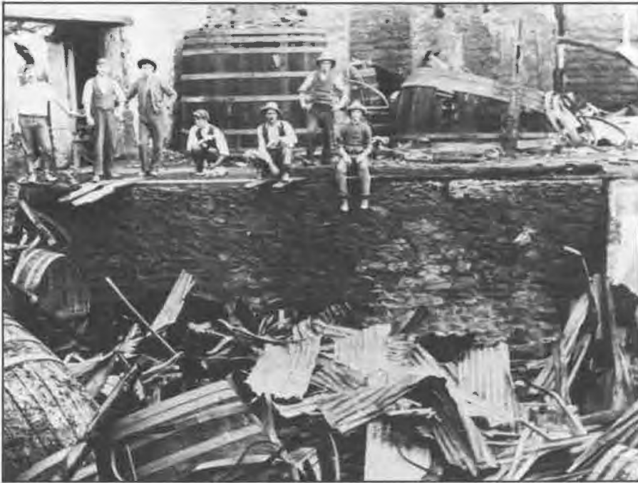
Damage caused by the fire at Bankside in 1904 (Thos. Hardy & Sons)
