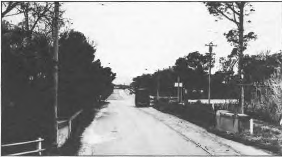
Henley Beach Road, before widening, looking to east (H.D.)
