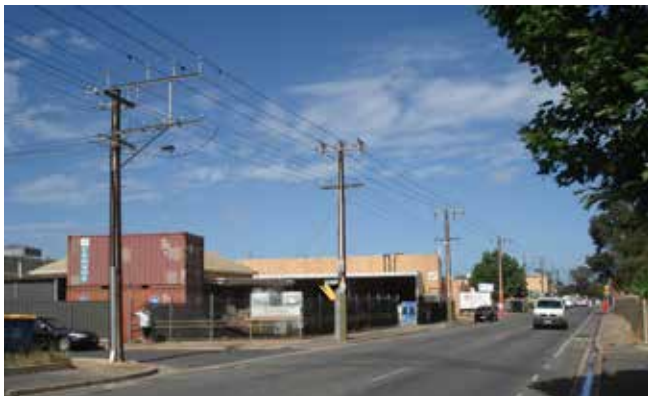
2.6.8 Varied building setback distances and off street car parking weaken the streetscape along West Thebarton Rd
