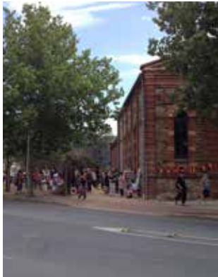
2.6.4 Former Church and Hall, on Phillips Street
