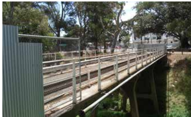
2.3.9 The closed tramway bridge at the end of Holland Street
