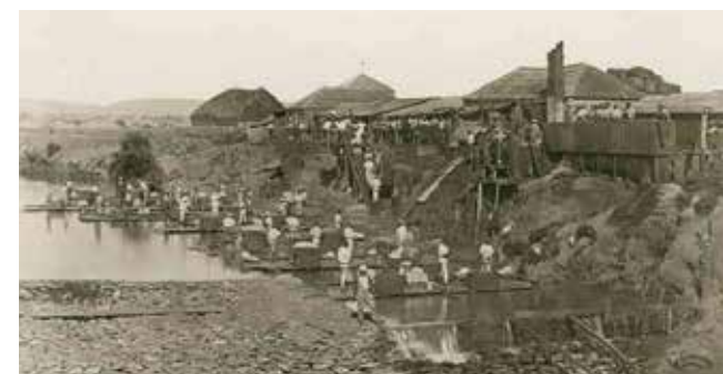
Damming of the River Torrens for wool washing
