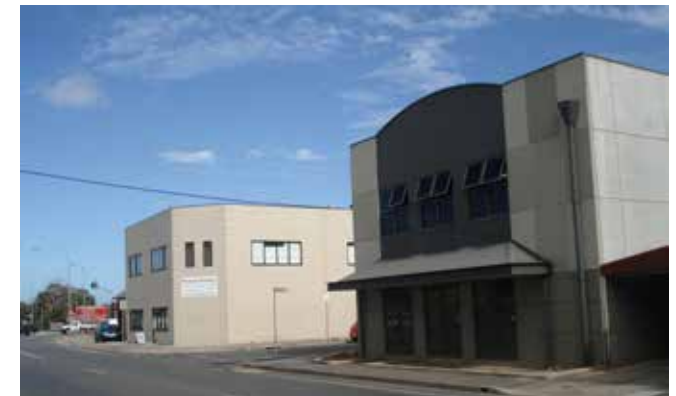
2.6.10 Non-active, poorly articulated facades fronting the street create a poor streetscape experience.
