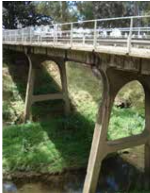
2.6.5 The Holland Street Tramway Bridge
