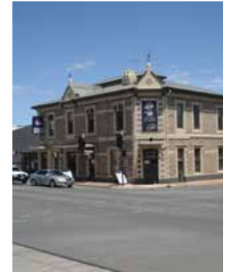
2.8.8 The Southwark Hotel on Port Rd/Phillips St
