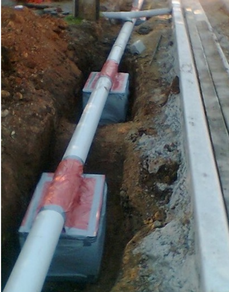
Stormwater 'Pod' (City of Burnside)
