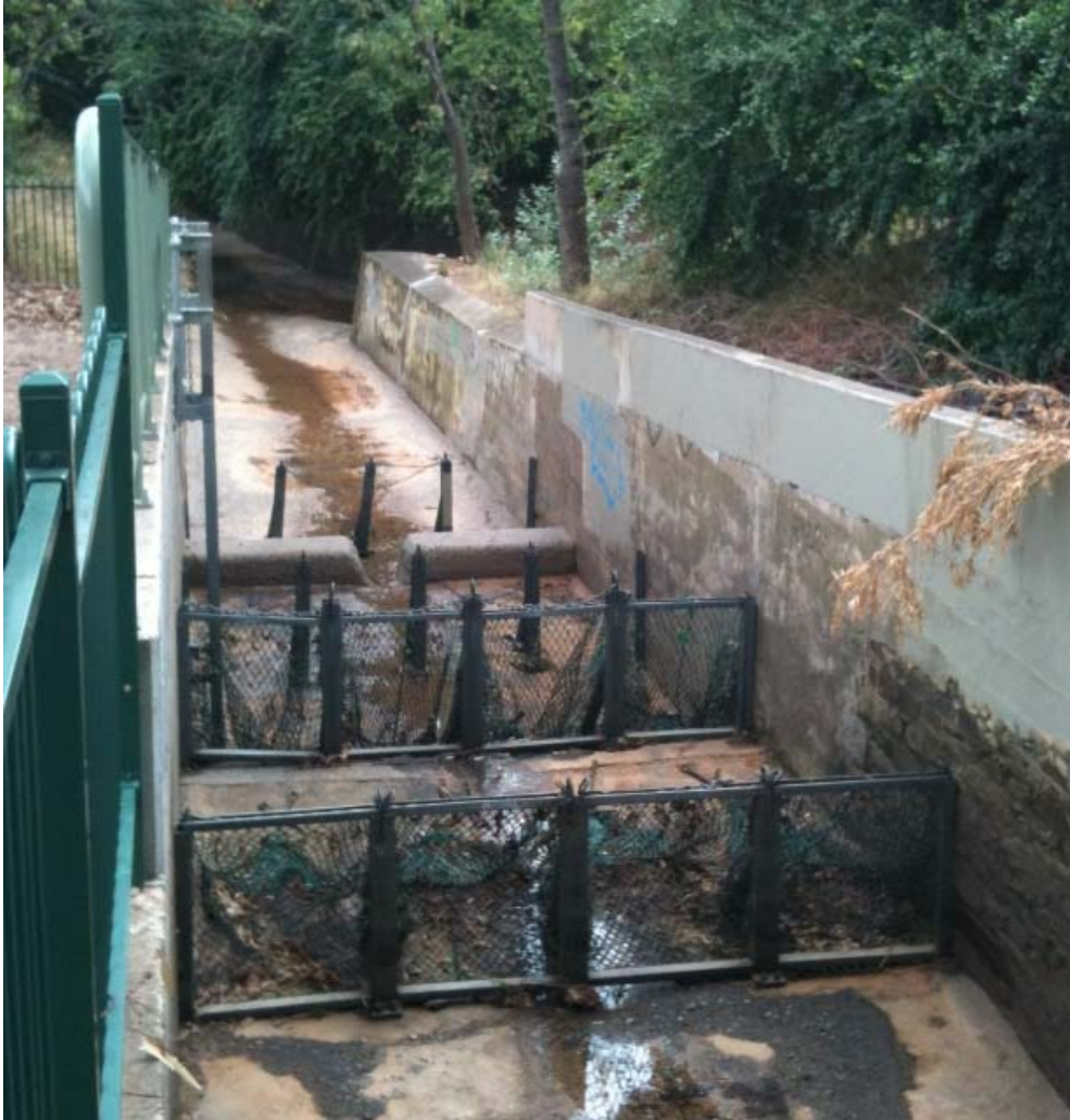
Glen Osmond Creek, Simpson Parade Trash Racks
