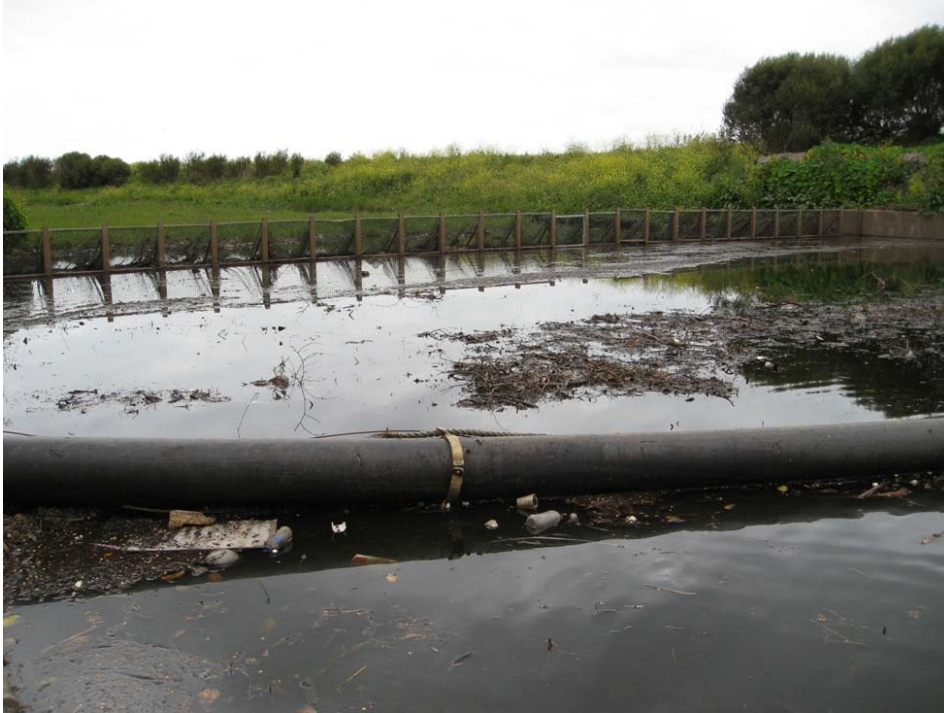
Brown Hill Creek, Watson Avenue Trash Rack, Floating Boom and Sediment Basin
