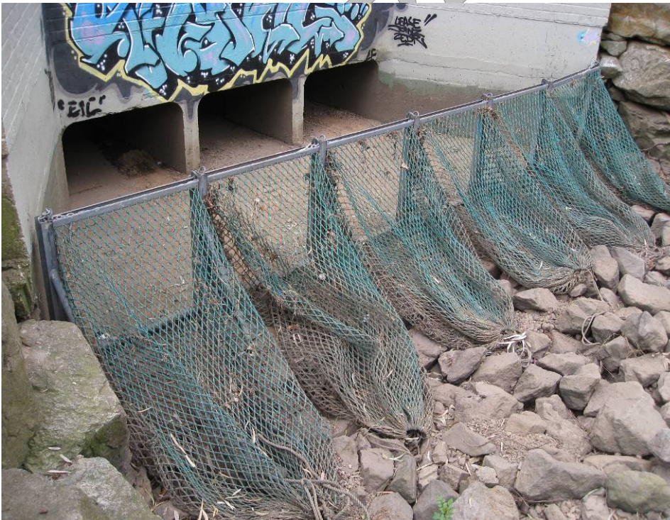
Parklands Creek, Park 20 Trash Rack
