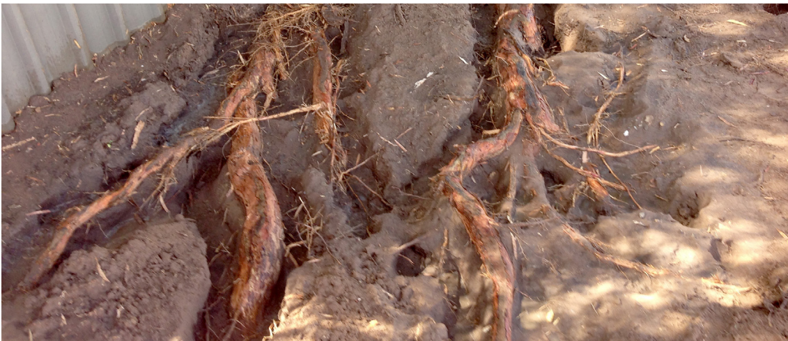
Tree root damage can be caused by established trees. This should be reported to Council by residents.
