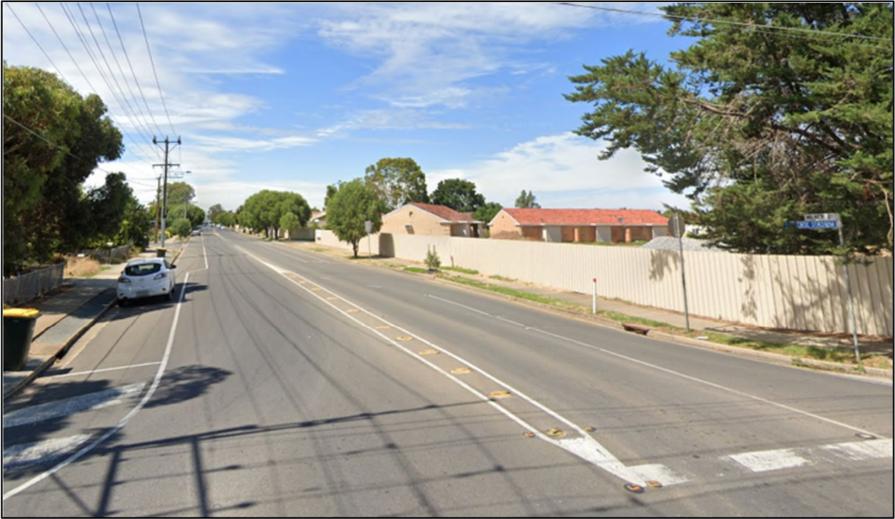
6.2.16 Pavement delineation Ebor Avenue/Halifax Street/Darebin Street.
