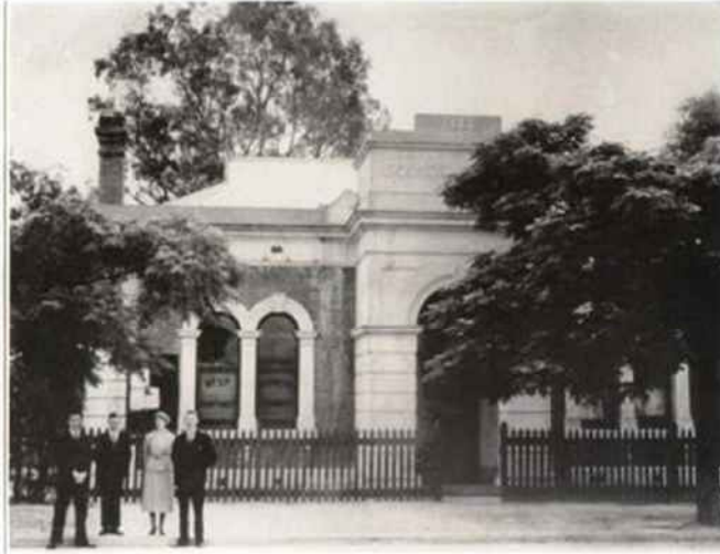
Figure 3: Photograph of Original Council Chambers Façade to Marion Road 1930 Source: City of West Torrens council records
