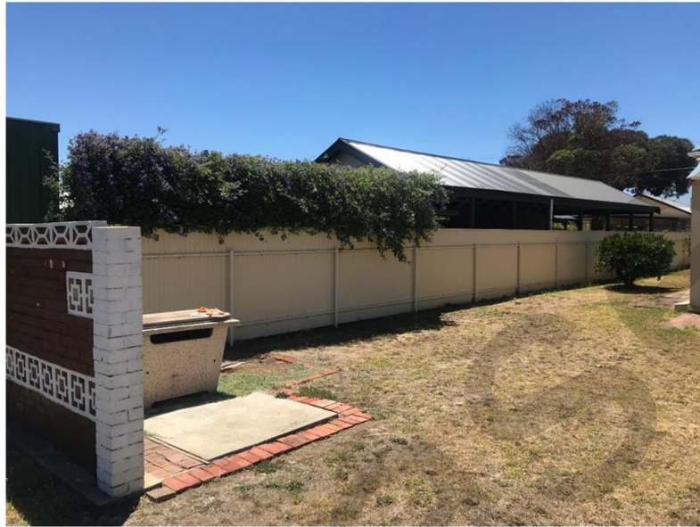
Photo 4: Existing fence along northern boundary.
