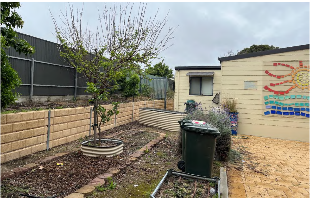
Figure 4: Existing retaining wall and fence along the southern boundary
