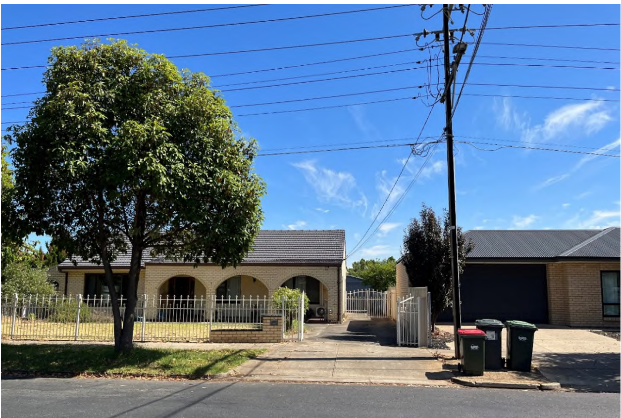
Figure 4: Subject land and adjoining dwelling to the east
