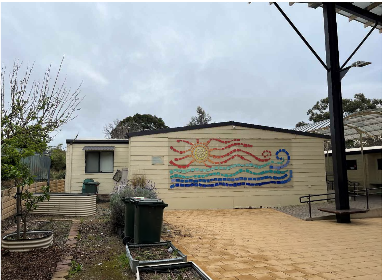
Figure 3: Existing Transportable Classrooms
