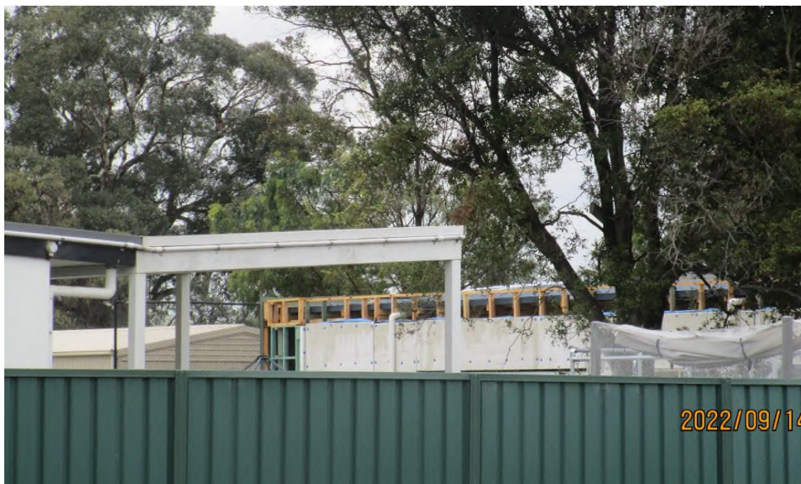
Figure 6 - Subject building, viewed from 27 Capper Street
