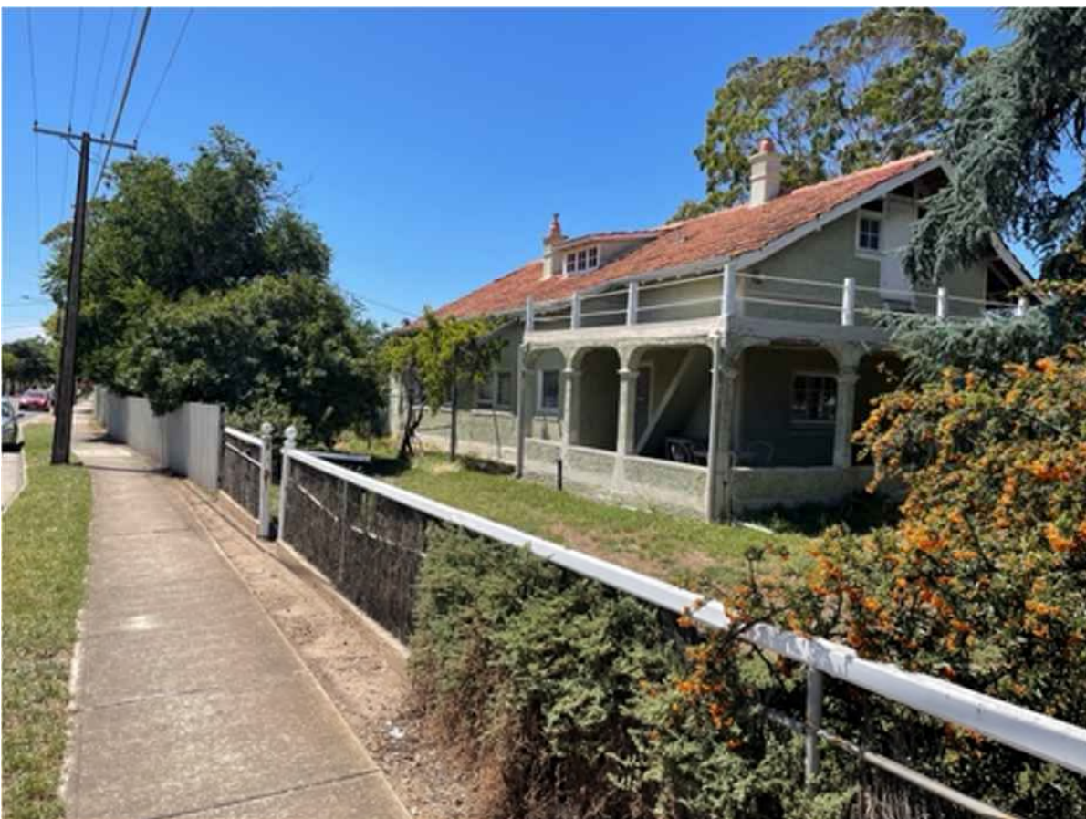
Figure 2 - Subject Site, western boundary, viewed towards the north (from Chambers Avenue)
