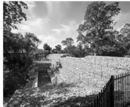
Flood Control Dam
