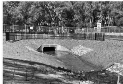
Park 20 new culvert and swale
