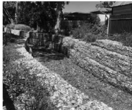
Rock filled gabions
