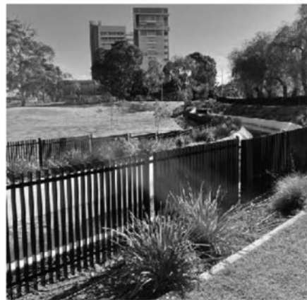
Concrete swale and fencing
