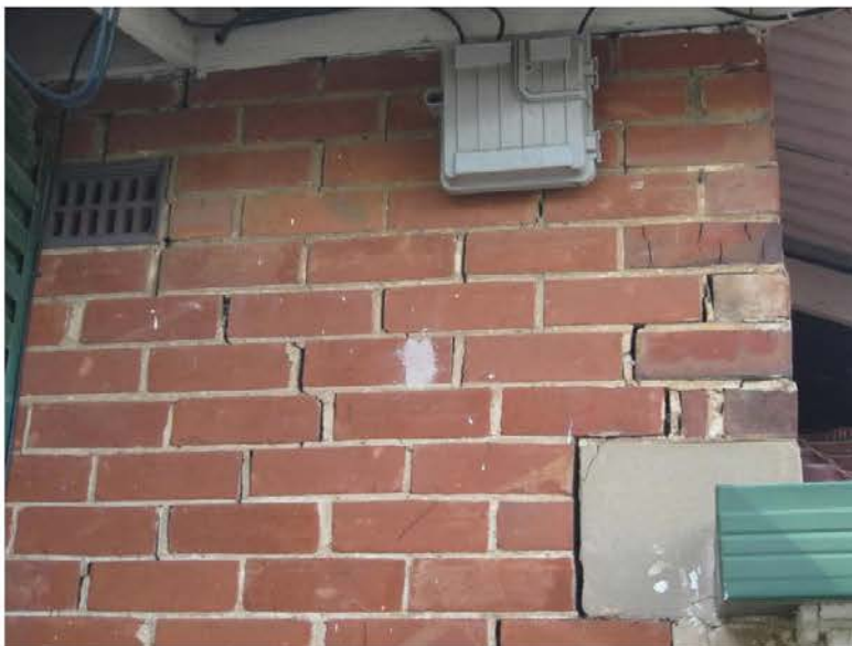
Cracking to the north western corner
