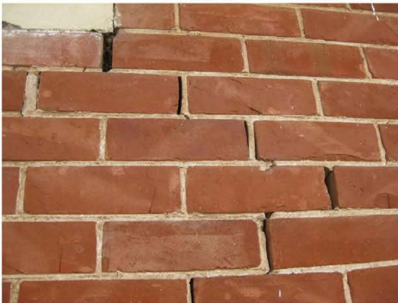
Cracking to southern external wall
