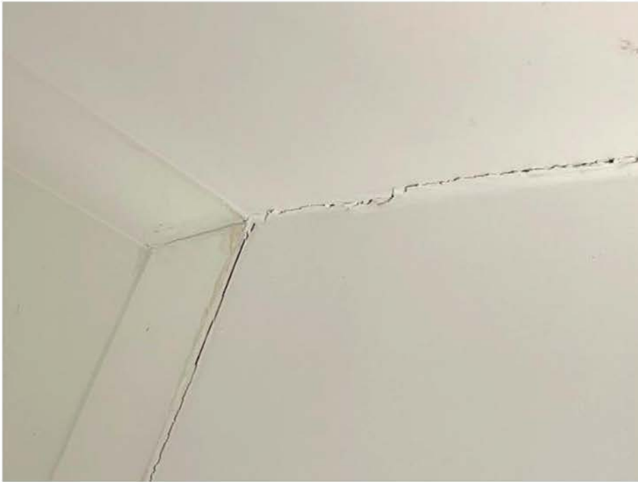
Figure 4 - Internal cracking to walls at 11 Clifford
