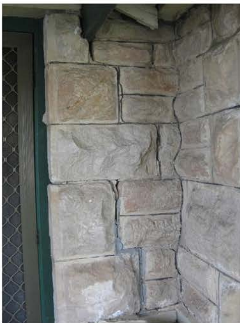
Crack next to front door
