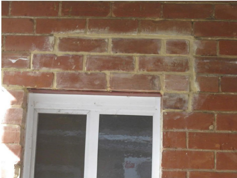
Patched crack to northern wall, closest to the tree
