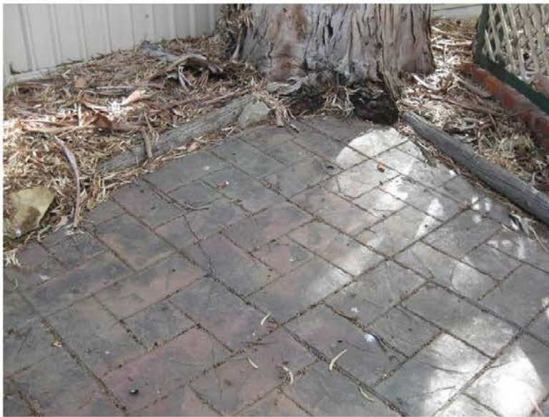
Cracks to paving next to the tree
