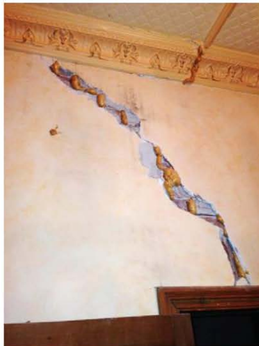
Figure 10 - Large internal cracking - 9 Clifford (Owner Provided)
