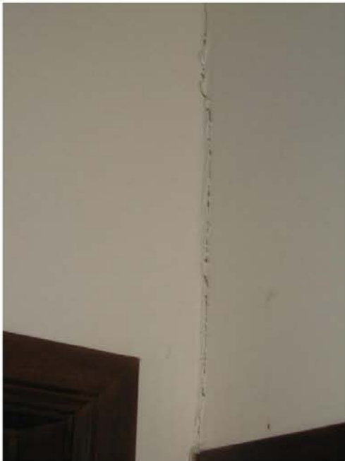
Cracking where the addition meets the original house
