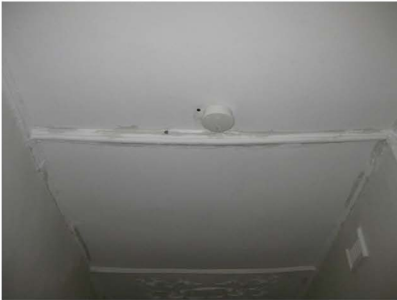
Cracking to ceiling in hallway
