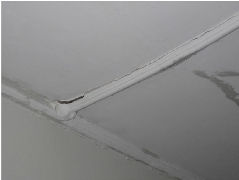
Cracking to ceiling front northern room
