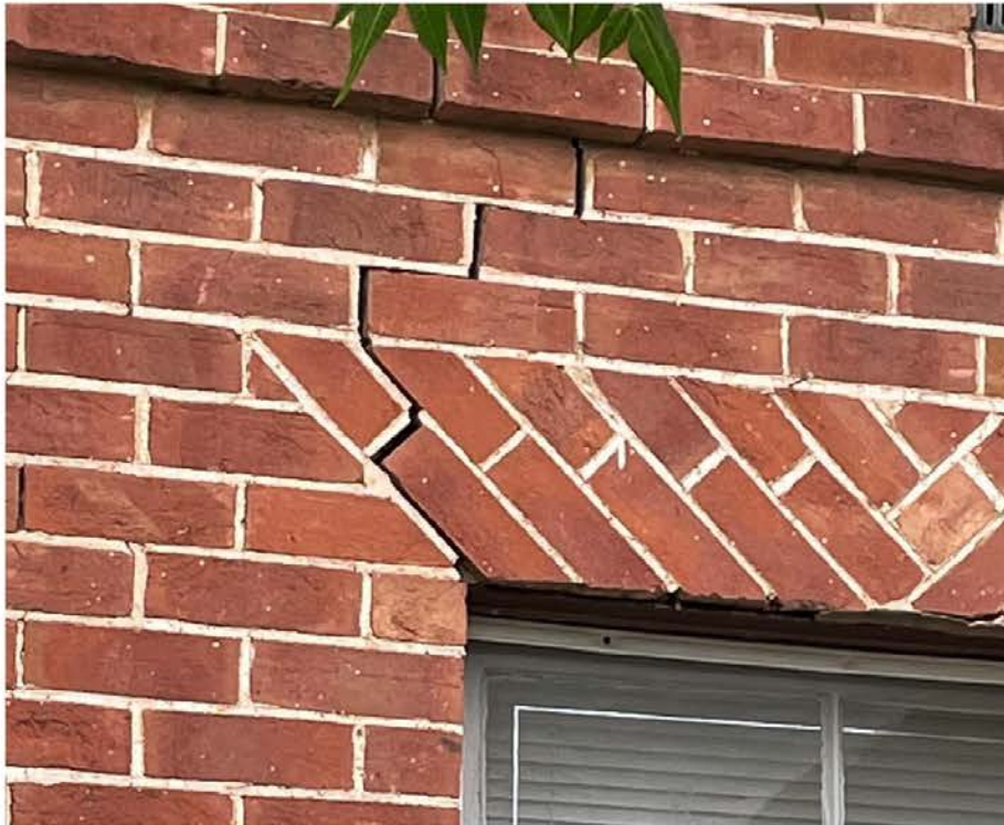
Figure 8 - 20+ mm wide crack at 9 Clifford
