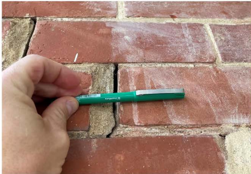
Figure 6 - Active crack at 11 Clifford
