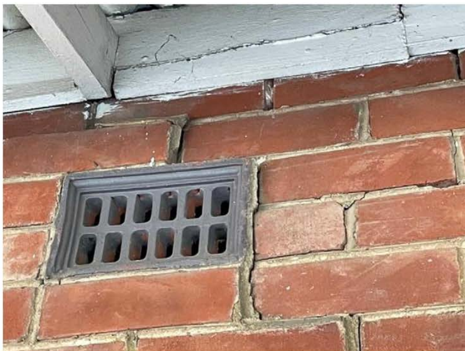
Figure 3 - Cracking and displacement of bricks at 11 Clifford
