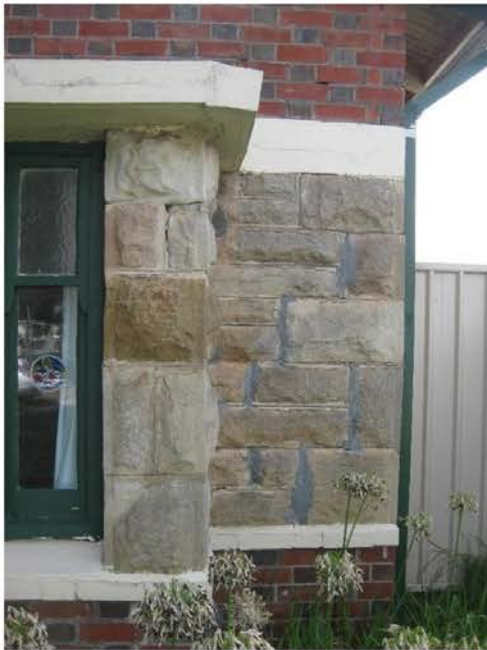
Patched crack to the southern end of the front western wall
