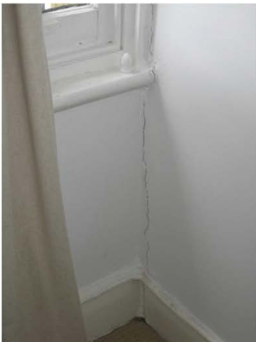
Cracking to front wall in the southern front room
