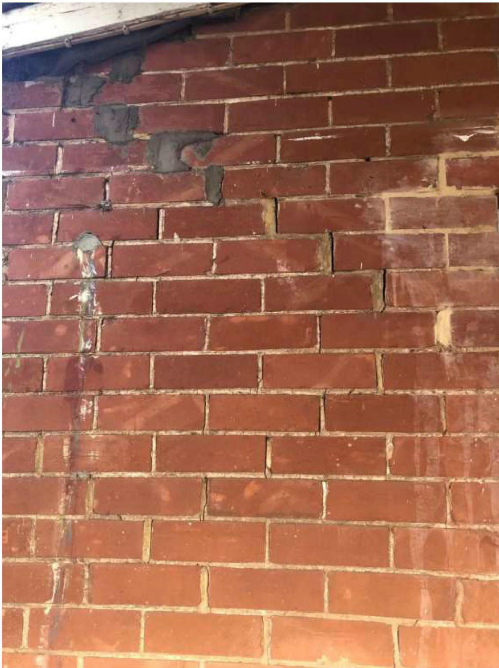
Figure 6: Cracked dwelling wall within the TPZ.
