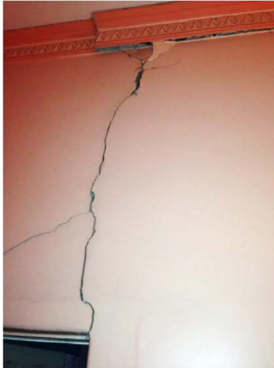
Figure 9 - Large cracking to internal wall - 9 Clifford (Owner Provided)
