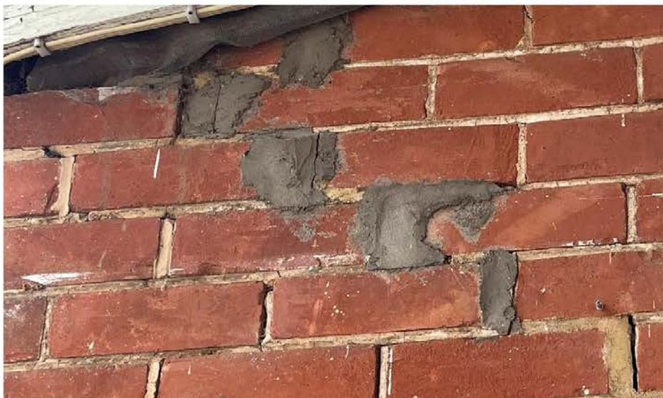
Figure 5 - Previously repaired wall crack reopening - 11 Clifford
