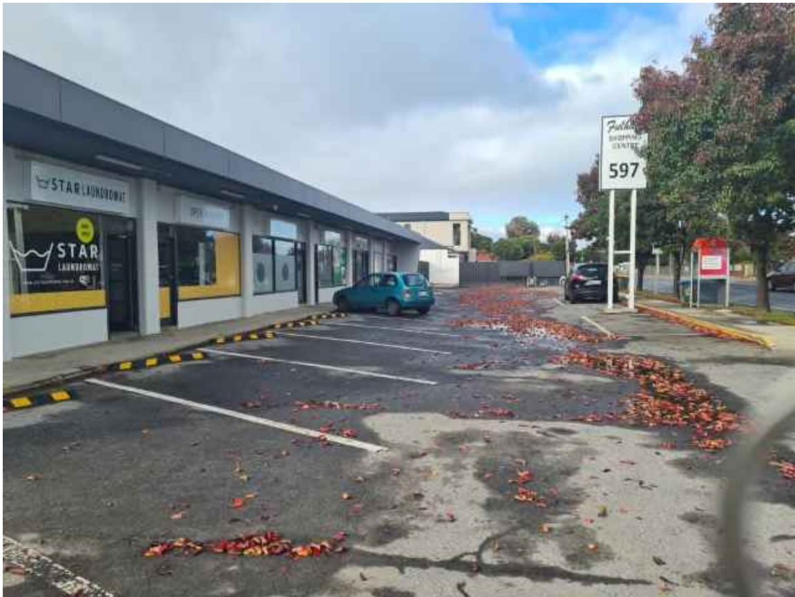
Figure 2: The subject group of shops viewed toward south
