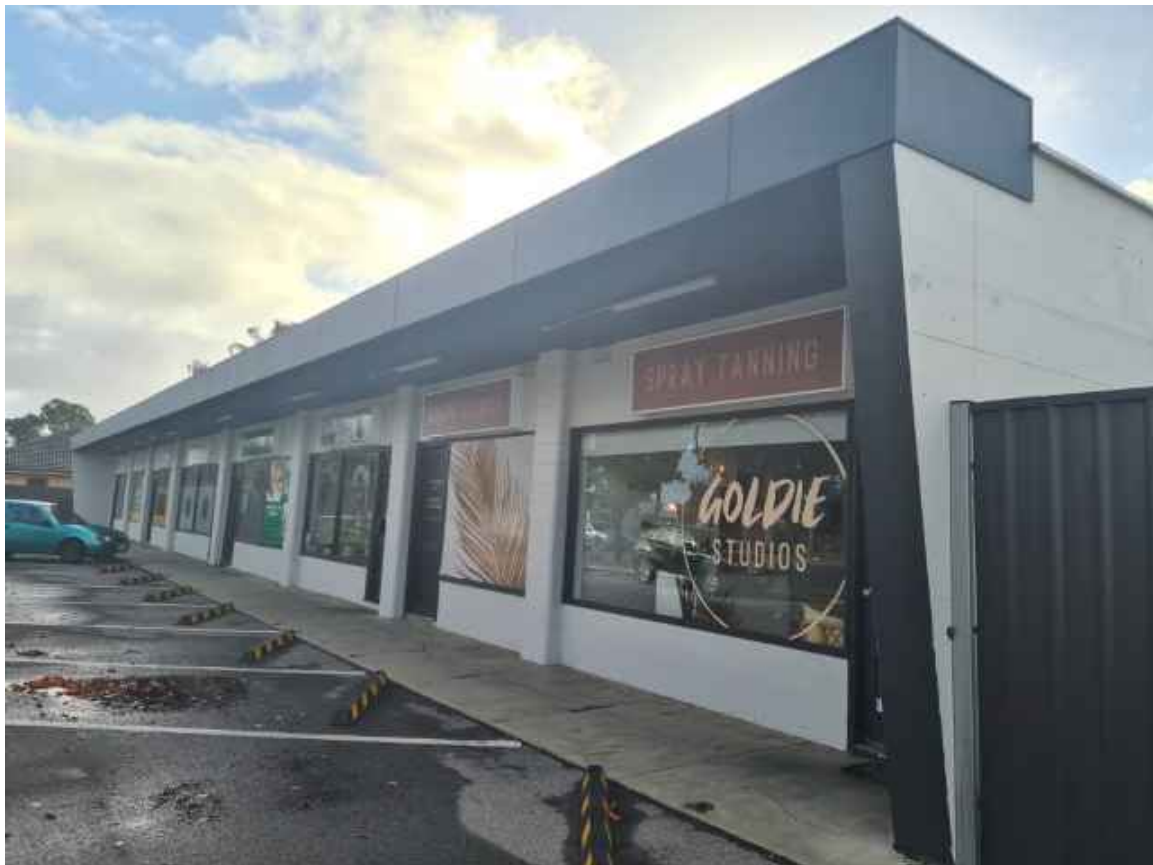
Figure 1: The subject land and group of shops viewed toward north
