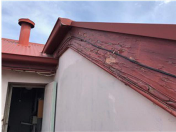
deteriorating timber
