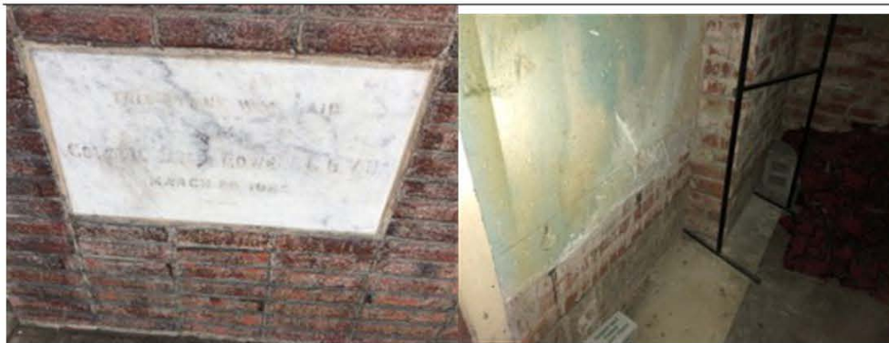
Foundation Stone from 1925 located in 1950's stack bond
