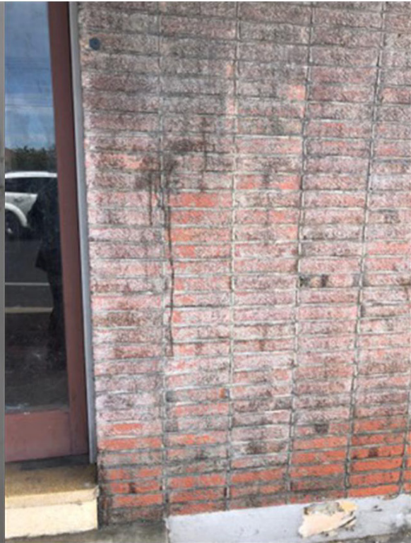
Detail of 1950's stack brickwork facing Henley Beach Road
