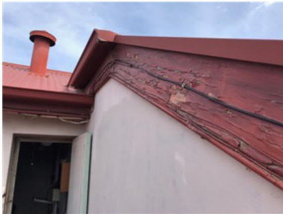
Possible, remnant front wall rendered over and deteriorating timber
