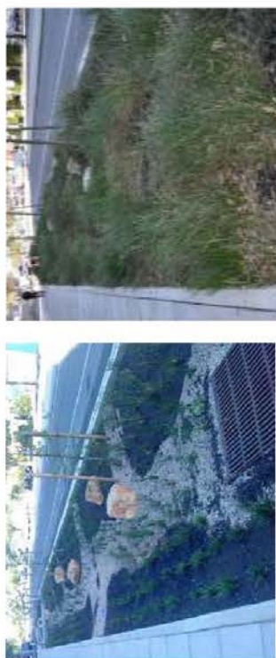
Angas Street, Adelaide raingarden (i) showing arrangement of filter media and (ii) once established.
