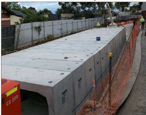
Culvert Installation
