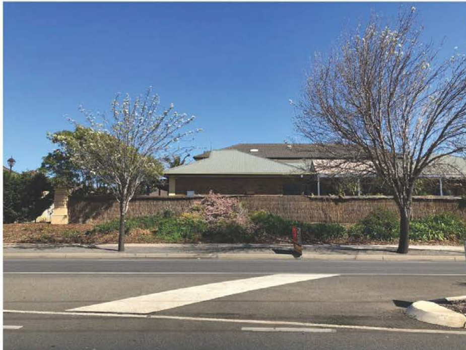
Figure 1: Fencing within the locality - 9 Ayliffe Place, Novar Gardens (subject site)
