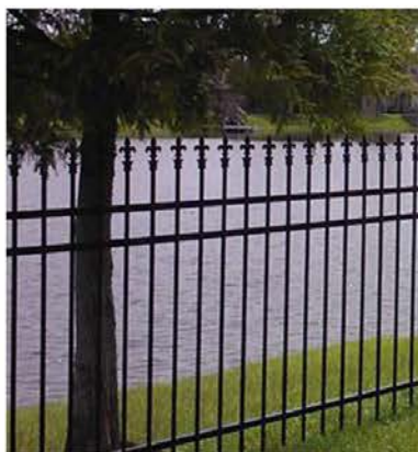
EXAMPLE - SQUARE HOLLOW SECTION FENCING IN STANDARD MODULES WITH 'FLEUR DE LIS' SPEAR TOP DETAIL
