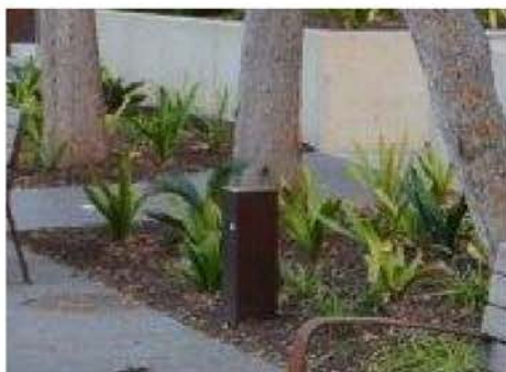
EXAMPLE OF POWER BOLLARD LOCATED WITHIN GARDEN BED
