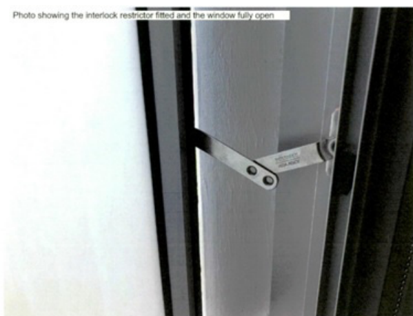
Image 3: View of window restrictor installed on each of the southern facing windows
