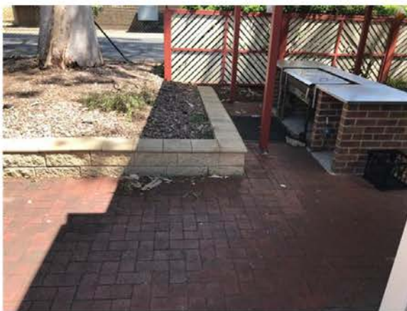
Showing the main stem emanating from the raised garden bed with only minor movement visible within the surrounding surfaces
