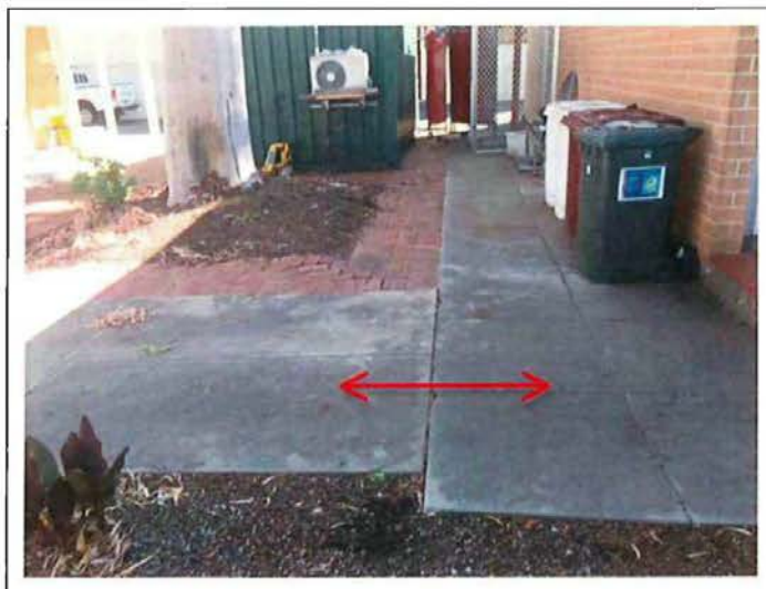
Figure 4 shows the hard surface area around the base of the Lemon Scented Gum Tree where it is proposed to remediate the area as a result of the unevenness caused by the subject tree. The arrow indicates an area of high traffic from employees at Arnott's.
