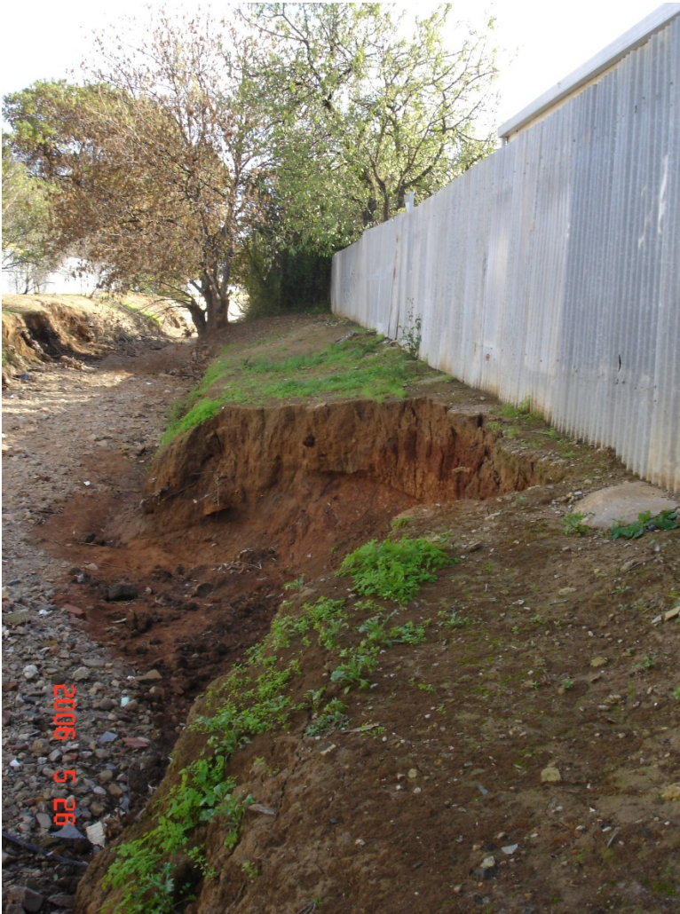
Photo 3: An example of explosive erosion, Brown Hill Creek
