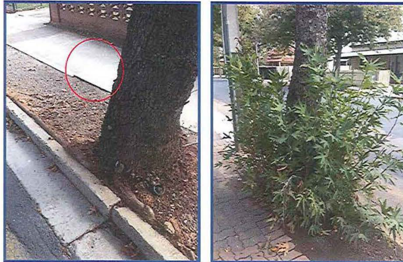
Figures 4 & 5: (Above left) the zone of rapid taper becomes damaging at an early age and its expansion does not stop until the tree matures. The red arrow indicates a trip hazard caused by the uplifting of the repaired sidewalk. Pavers are more ideal in this situation as they 're-set' several times to roll over the expanding root system. This system has already been implemented on the southern side of George Street. (Above right) provides an image of a mass of epicormic growth emanating from the base of a subject tree. This indicates that some trees are struggling with their restrictive growing conditions.
